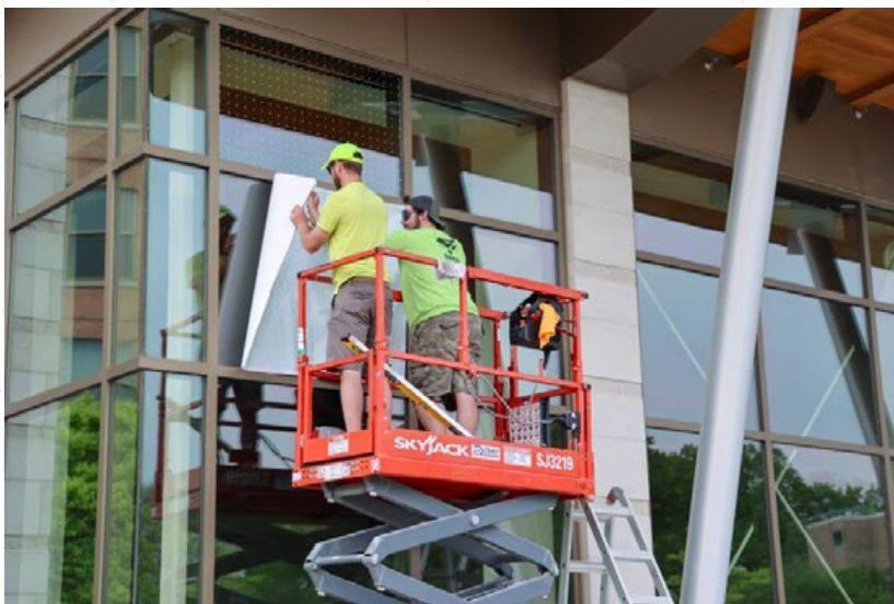
Two workers install window dots as part of the bird-friendly glass Green Fund project. Photos by Lauren Graves (4)
