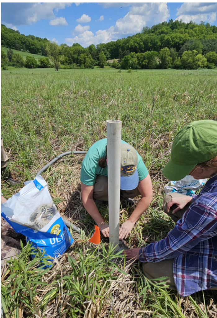
Van Alsburg’s team installs a groundwater well.
