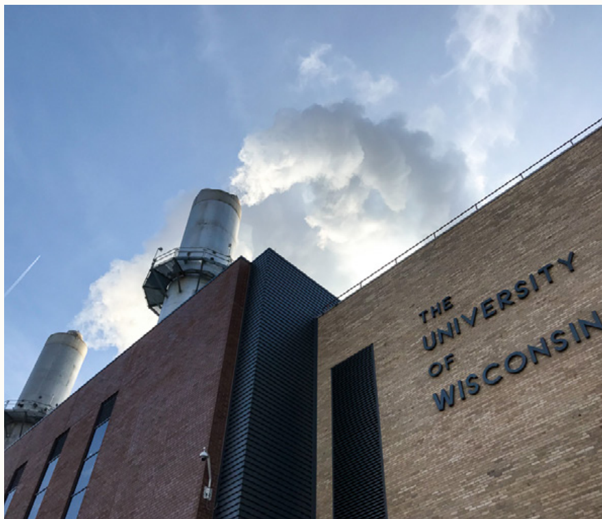
The Charter Street Heating & Cooling Plant at UW–Madison runs on natural gas and provides steam and chilled water to campus buildings. Photo by Nathan Jandl
